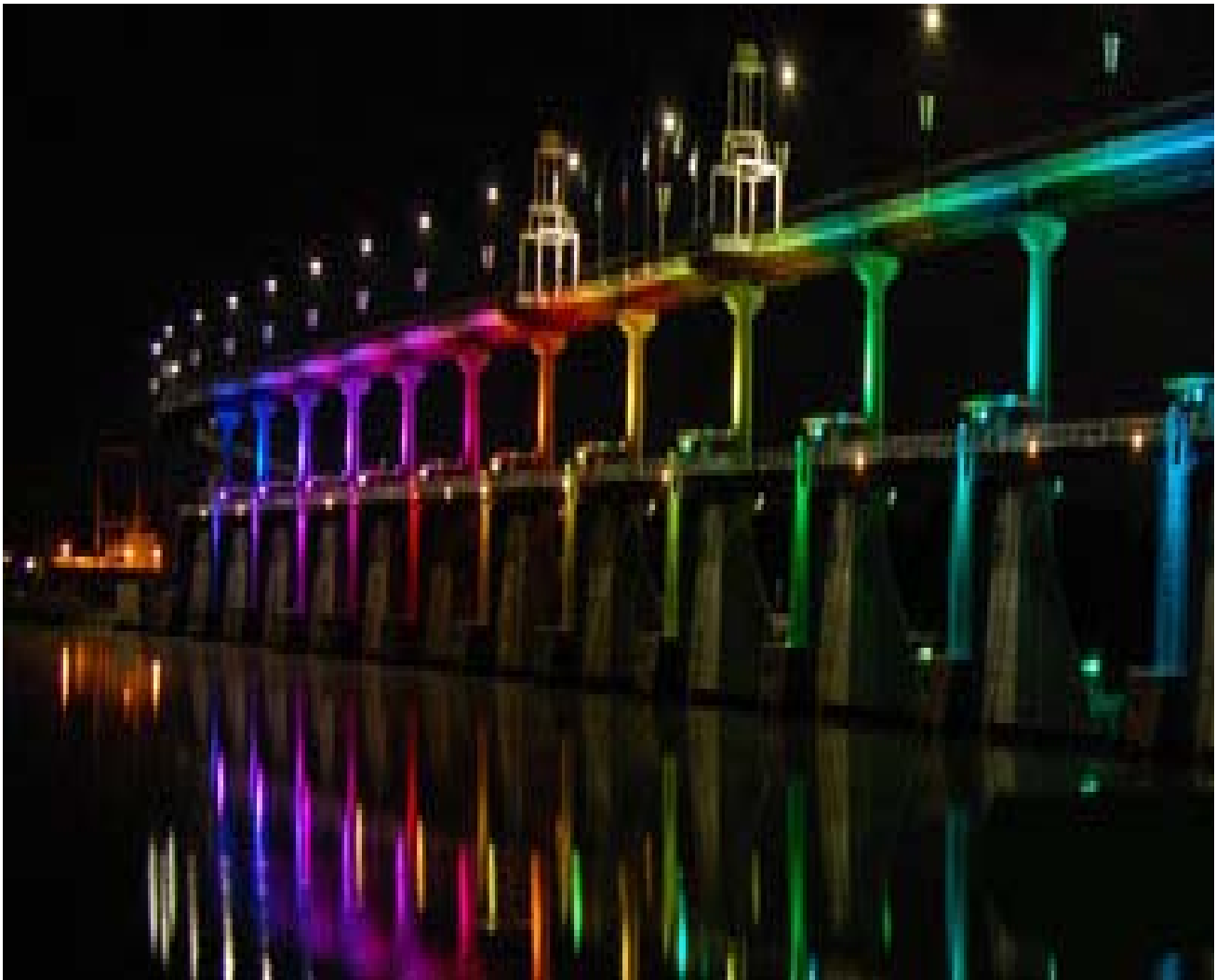
BIG DAM BRIDGE
